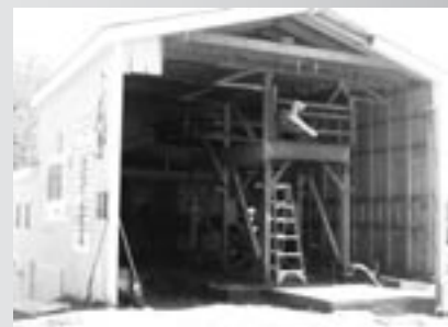
The building around the drive station will be re-used, the components will be removed and the "Crows Nest" will be restored to its original greatness.
